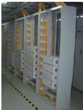
Optical distribution frame
