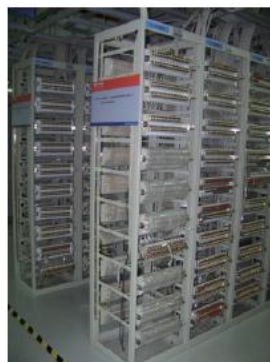
Digital distribution frame
