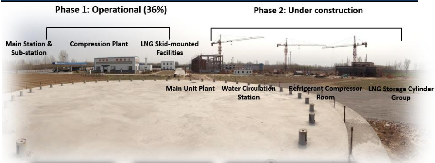
Figure 4: Construction site for expansion of Shandong project
