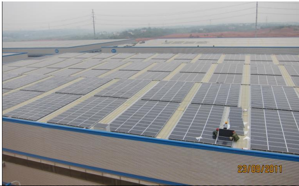
Photo set 2. Hunan factory 20MW Roof-top under "Golden Sun Project"
