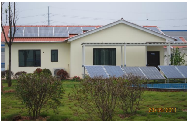
Photo set 3. Solar house demonstration in Hunan
