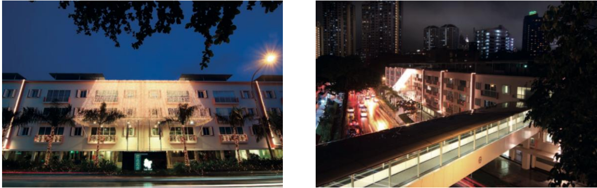
Figure 2. Link Hotel (left) and Link Bridge (right)
