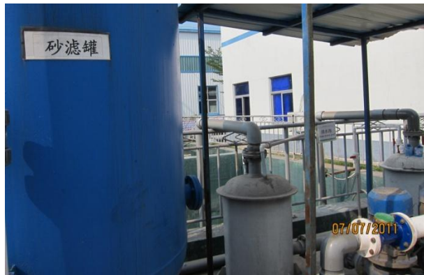
Photo set 1. Waste water treatment at Zhaoqing plant
